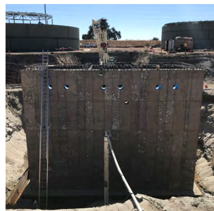
The newly poured pumping station measures 40 feet tall x 36 long x 12 feet wide. Concrete treated with Xypex Bio-San C500 Admix provides complete protection from water ingress, sewage exfiltration, and microbial induced corrosion.
